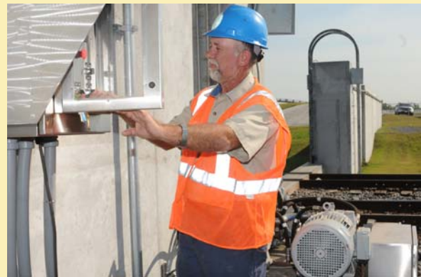
Bart LeBlanc, PLD Maintenance Shop Superintendent, pushes the buttons to close the railroad swing gate during hurricane exercises on May 15. The gate closed flawlessly.
