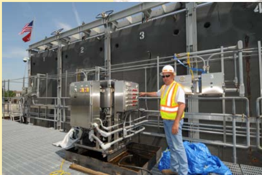
Corps operator Stacey Hodnett, left, mans the controls to close the gates at the Orleans Ave. Outfall Canal.
